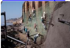
Colton Seawall Under Construction
