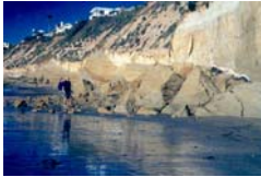
Solana Beach Sea Cliff Collapse
