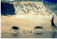
Dec. 1997, Blackburn Slope Failure
