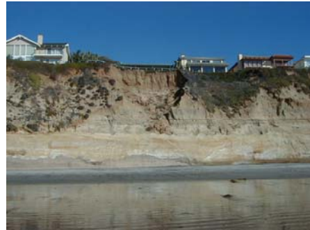
36 Bluff Failures in the Last 36 Months
